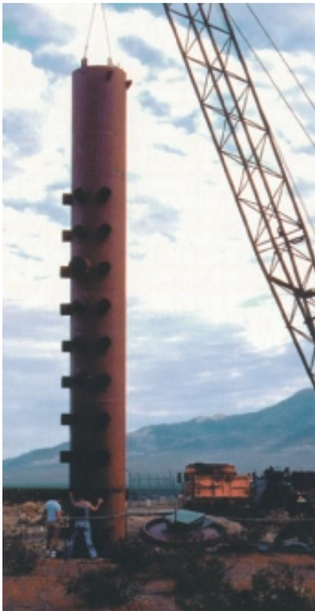
Vertical shaft (5 feet in diameter and 45 feet deep) installed at the Amargosa Desert Research Site provides access to measure movement of moisture and contaminants in the dry zone above the water table.
